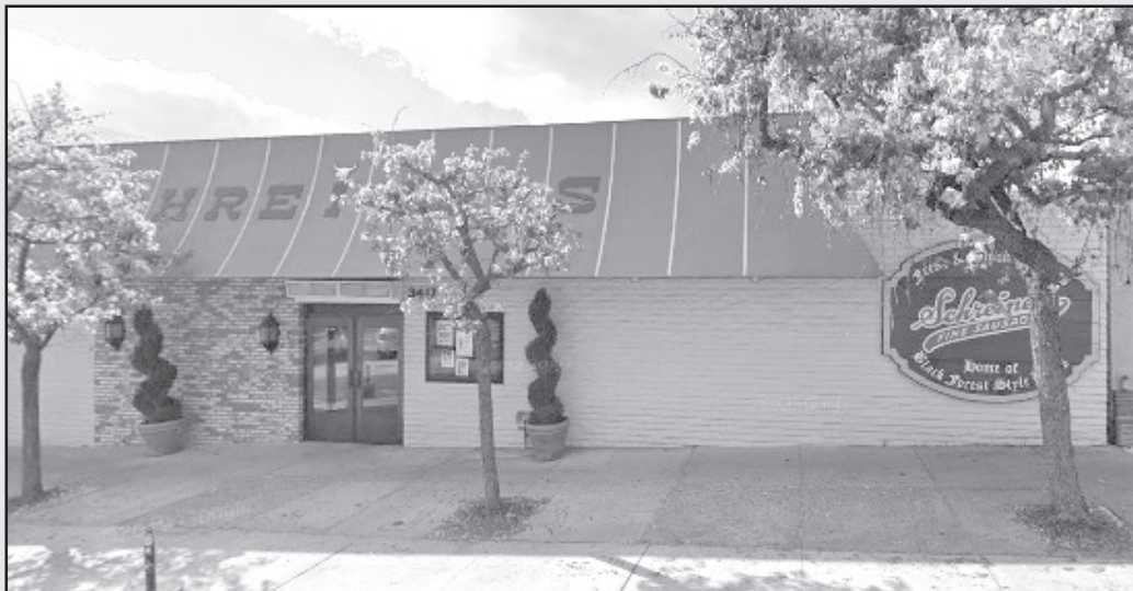
Now » In 1952 Schreiner's Fine Sausages moved into the little building at 3417 Ocean View. Three generations of Schreiners have run the German food shop and in the process built a larger building.
