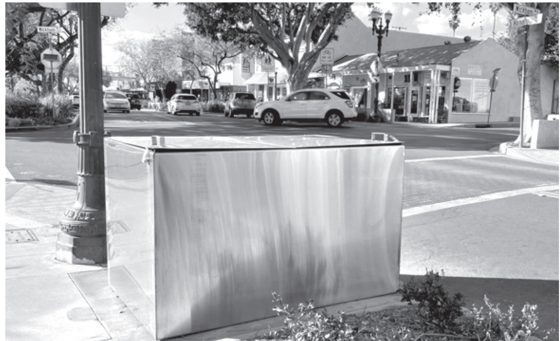
Photo by Mary O'KEEFE Silver boxes found on Honolulu Avenue house a barricade system that is unusable.
