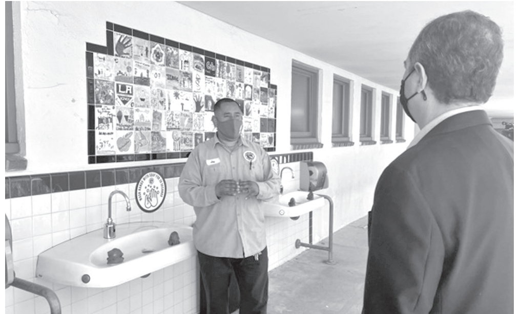
Photo by Mary O'KEEFE At Balboa Elementary School, custodian Jasen Laca explains to Congressman Adam Schiff the dual purpose of the hand-washing and water bottle filling stations.
