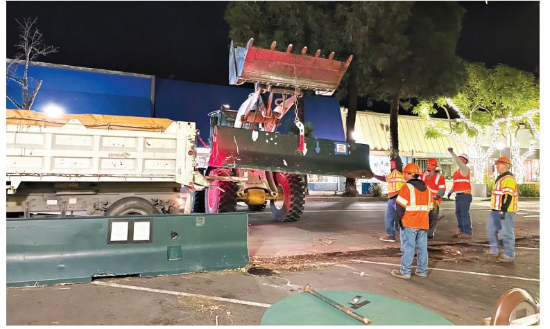
Photo by Mary O’KEEFE In the early morning hours of Oct. 14, the K-rails were removed from Honolulu Avenue. Glendale City Council has approved the design – and funding – for replacements.
