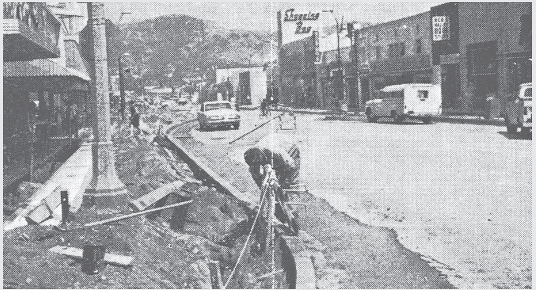
THEN: This newspaper photo from June 1967 shows the new curbing being finished for the soon-to-open Montrose Shopping Park. We're looking east down Honolulu Avenue from Ocean View Boulevard.
