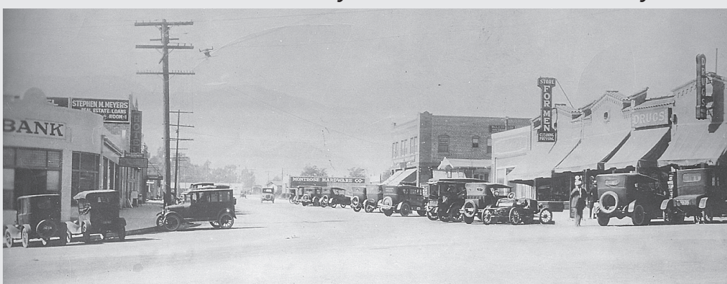
THEN: This was a busy Montrose in 1925. The view is looking west on Honolulu Avenue from its intersection with Verdugo. The street is wide and bare, its main feature being the telephone poles. Most of the buildings shown here are still standing.
