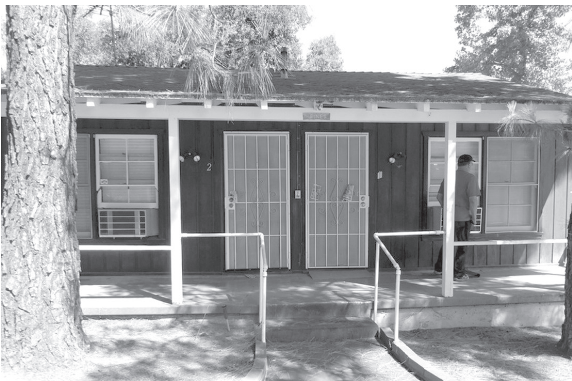
File photo Buildings on the Twelve Oaks Senior Living property, including the individual bungalows, are expected to be torn down as part of a complete remodel.
